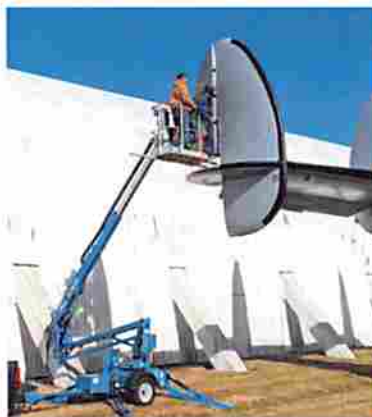
Welch and Madden install a rudder (K. Drewelow photo)
